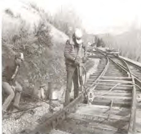
Laying track. Daun Bohall photo
