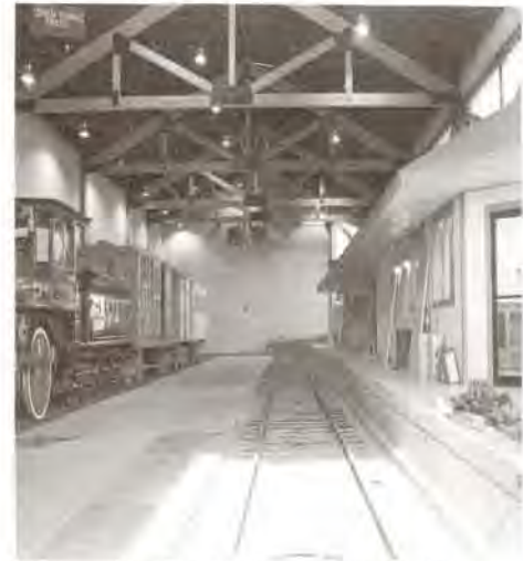
Interpretive Center nears completion, January 1990. Daun Bohall photo
