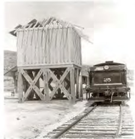
Water tower under construction. Daun Bohall photo
