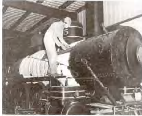
New insulation for #25. Daun Bohall photo
