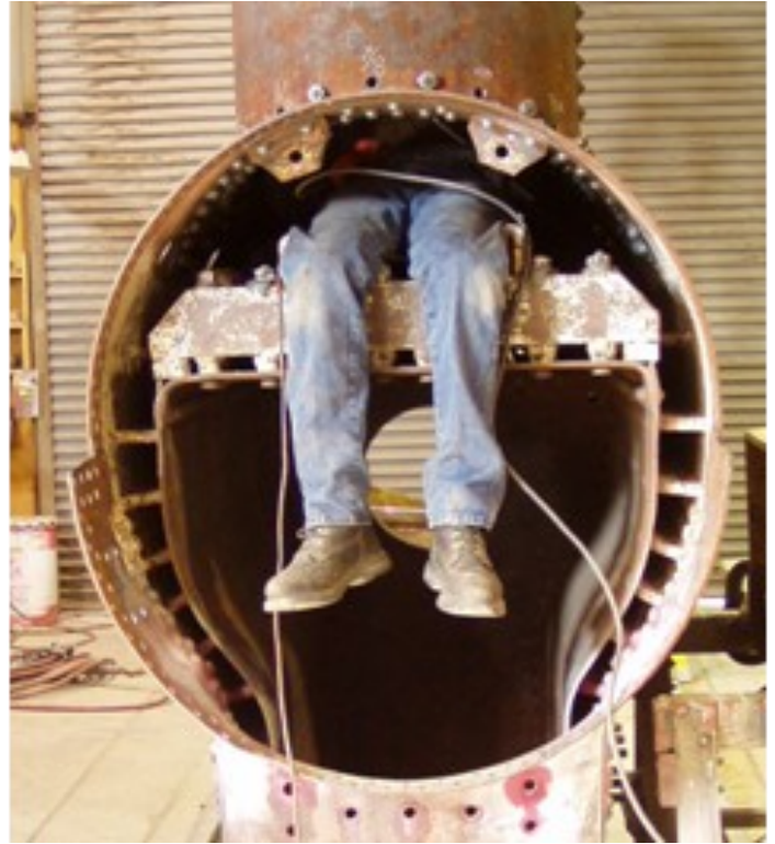
Volunteer Kevin Owens prepares the steam dome for riveting. November 2011
