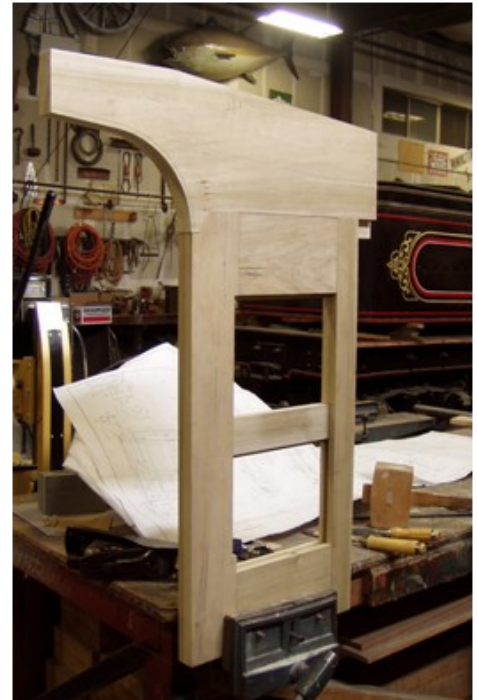
A mock-up of a rear cab-wall helps with joint design and layout. February 2012
