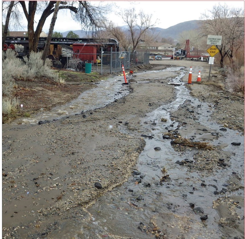
Flood waters and silt destroyed the rear entrance road of the museum, which limited access in the event of an emergency.
